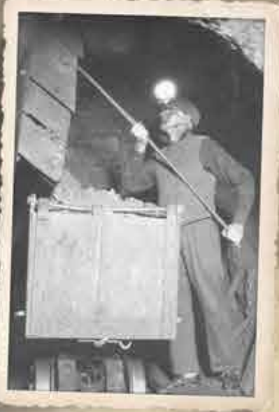
Cleaning out an ore chute into the underground tram, around 1937 ETHEL LECOUNT COLLECTION, COURTESY OF JEAN REPLINGER, MARSHALL, MN
