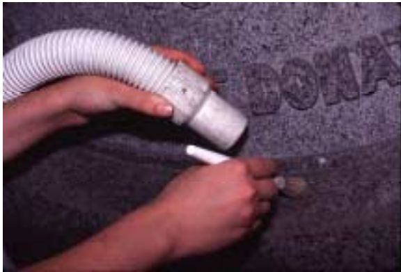
Figure 2. Vacuum cleaner dusting with a stencil brush.
