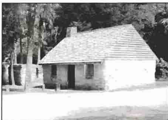
Figure 17. Restored Cabin E1.
