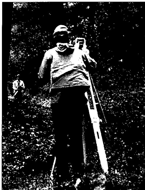
Figure 4. Surveyors using laser transits to perform a topographic survey. San Juan National Historical Park. (NPS, 1987)
