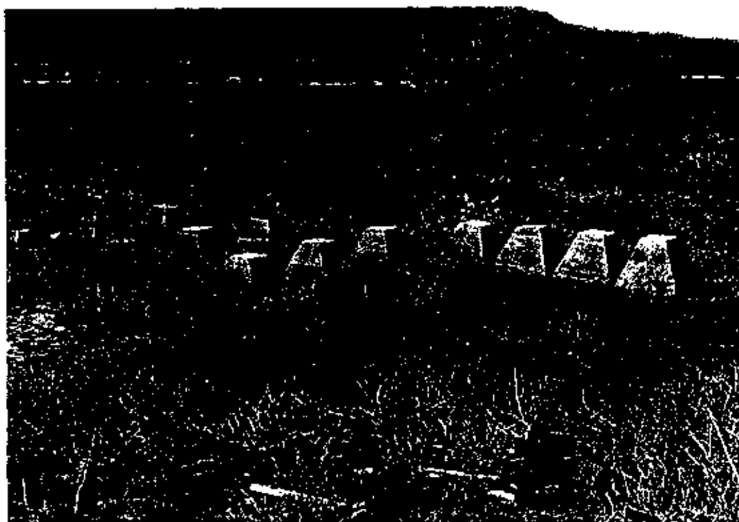
Figure 37. Concrete pier supports for former oil-drum loading ramp (Feature 6), from northeast, September, 1999. Photograph: William Chapman.
