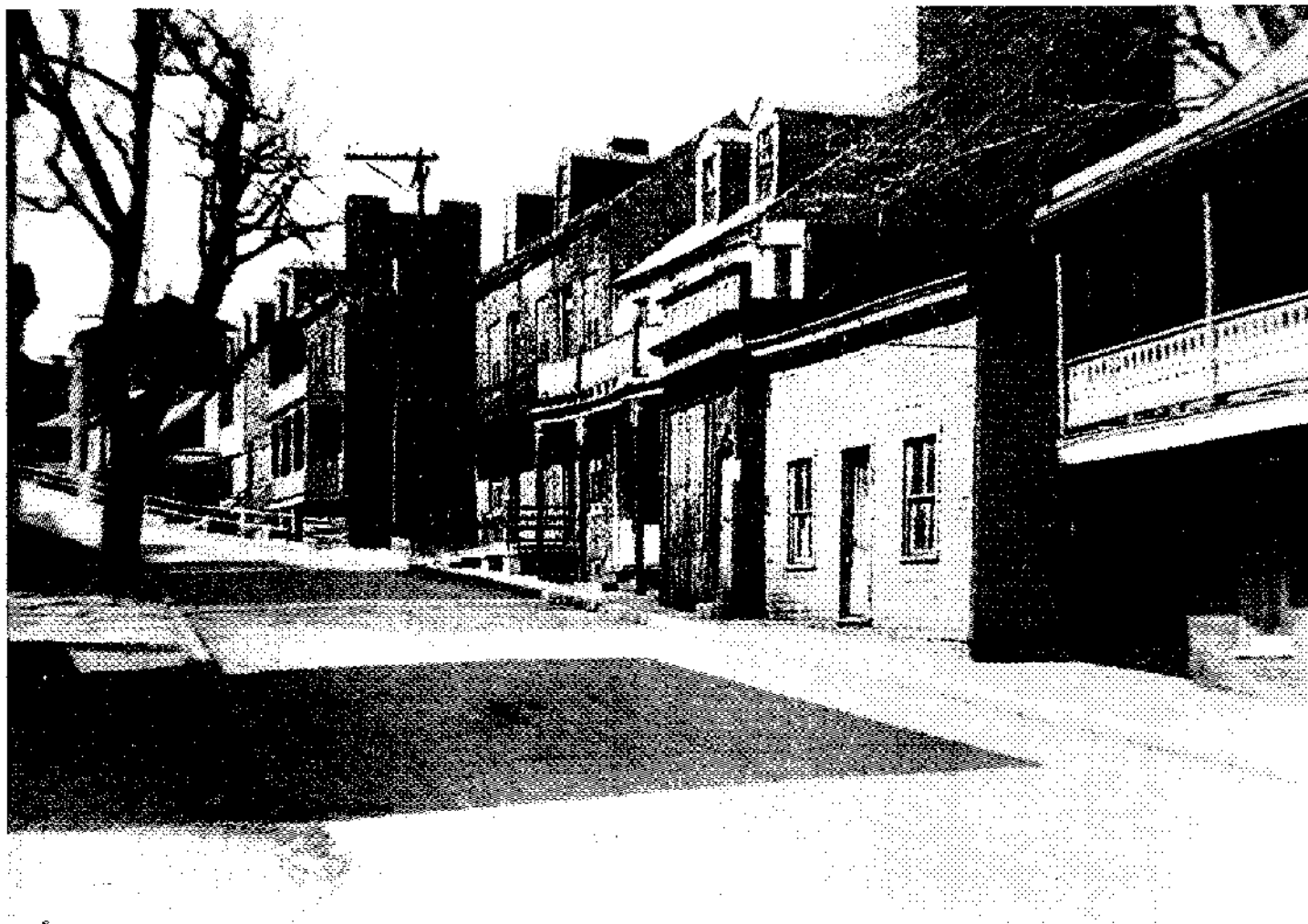
Fig. 14: High Street, Partly park and privately owned buildings, park buildings 12a, 13, 14, 15, and 16, 1955. Gift of Ames W. Williams 1979 (NHF 3860, Harpers Ferry NHP).
