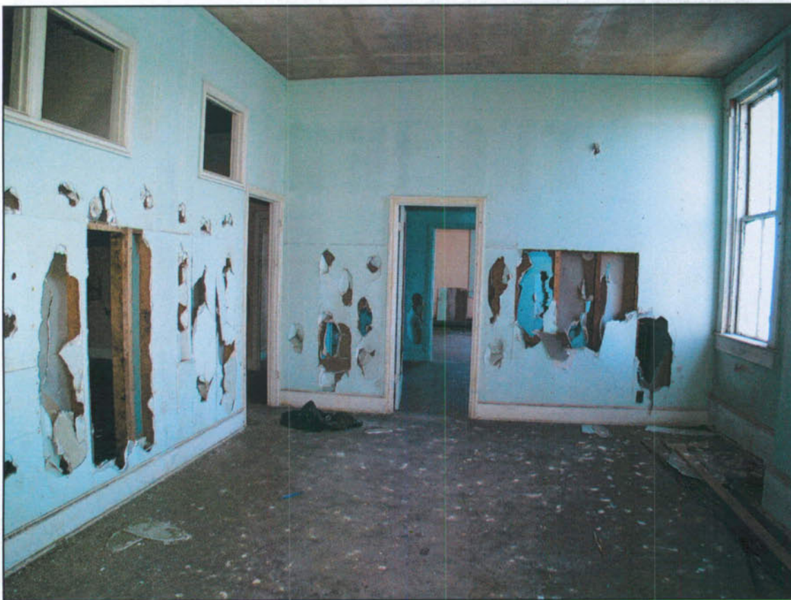
Above: Typical apartment interior with 1/4" gypsum board partition walls, 2003. Photo Credit: John Martini.
