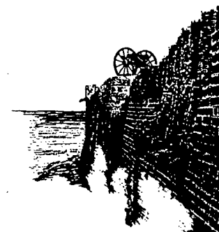
GABIONS USED TO SHORE UP WALLS.
