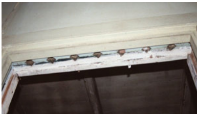
Evidence of original bars Window 11, Room 103
