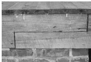
FIGURE 16. Left, detail of corner joint at corner of gallery; right, detail of lap joint in sill beams.
