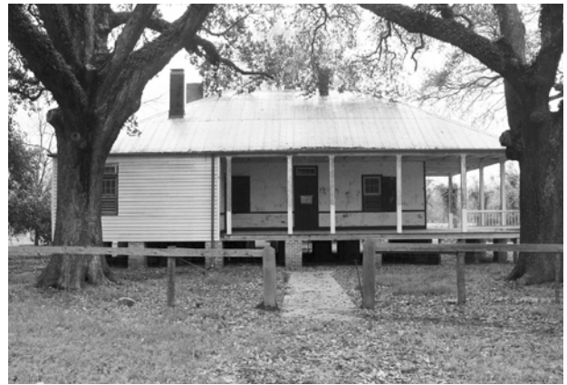
FIGURE 1. Southwest elevation, front entrance to Overseer's House.
