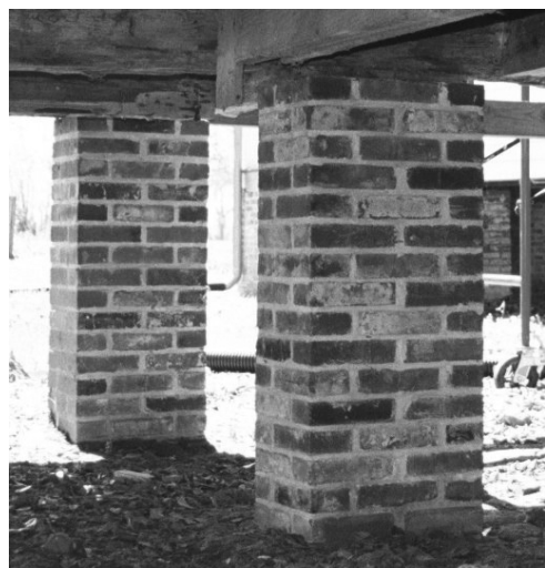
FIGURE 3. Foundation piers beneath Room 111 addition.
