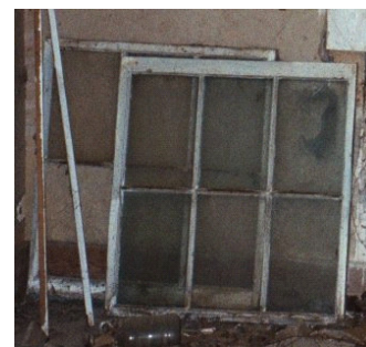
Sashes stored in Room 111, possibly from Window 15
