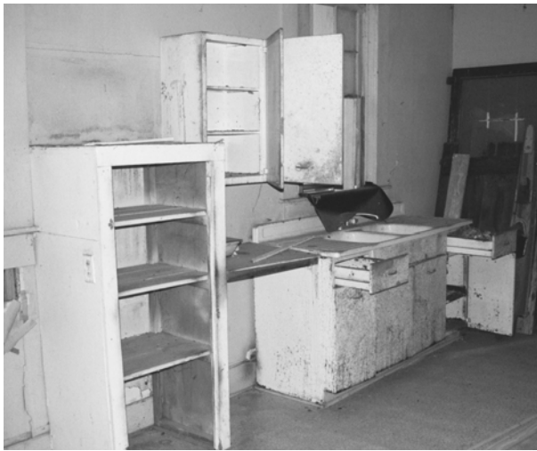
FIGURE 56. Cabinets and sink in Room 105.
