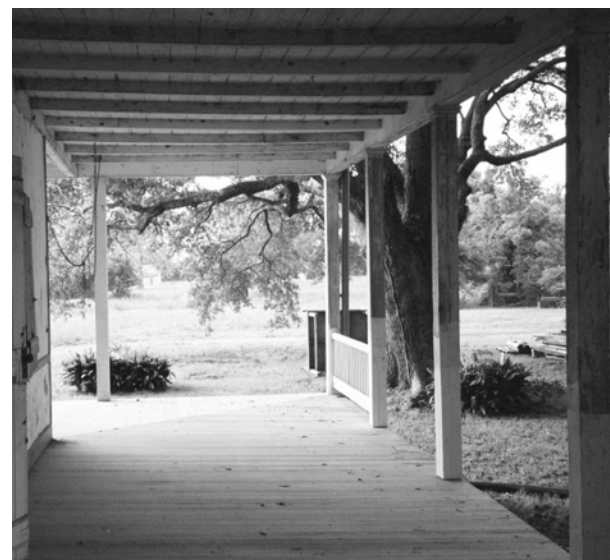
FIGURE 22. Southwest gallery looking southeast.
