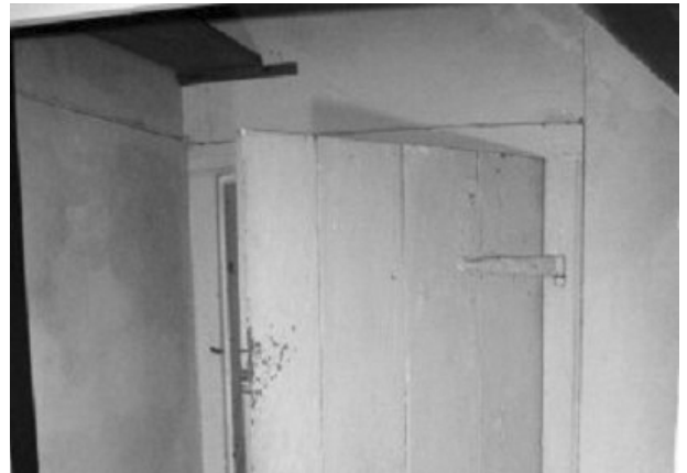
FIGURE 60. Room 107, note shelf on southwest wall.
