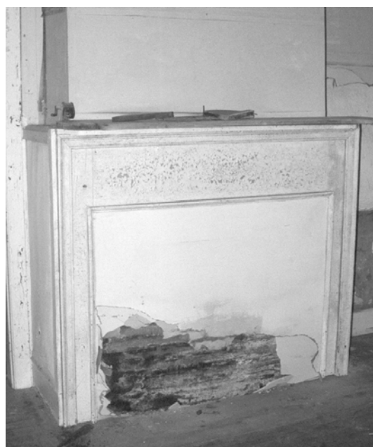
FIGURE 55. Fireplace #2 in Room 103.
