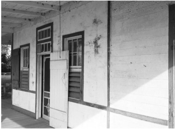
FIGURE 29. Southwest exterior walls at Rooms 104 and 105.
