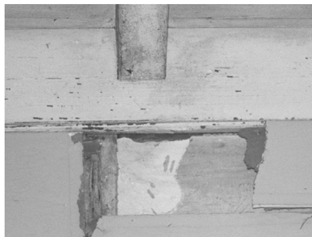
FIGURE 53. Room 104, ceiling joist (note bead), beam and exposed bousillage beneath gypsum wallboard.
