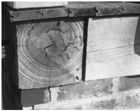
FIGURE 16. Left, detail of corner joint at corner of gallery; right, detail of lap joint in sill beams.
