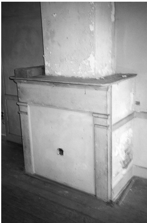
FIGURE 43. Fireplace #4 in Room 101.
