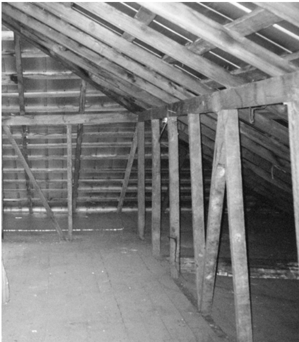
FIGURE 24. Knee walls in attic, looking northwest.
