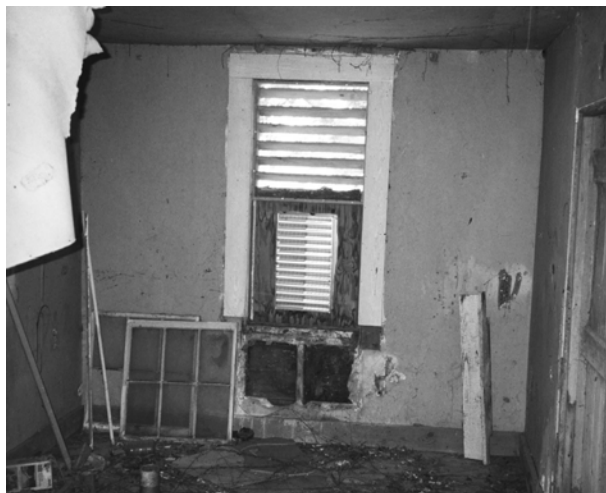
FIGURE 67. Northeast wall, Room 111.
