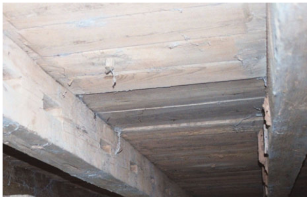
FIGURE 15. Above, pegged connections in historic floor framing; below, recycled joist in northwestern section of floor framing.
