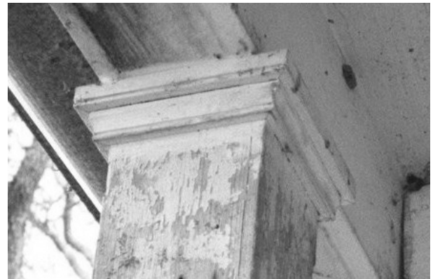
FIGURE 27. Typical column capital.
