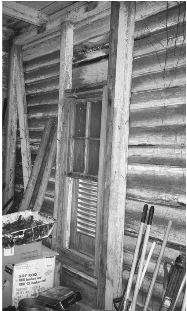
FIGURE 65. Northwest wall, Room 110.
