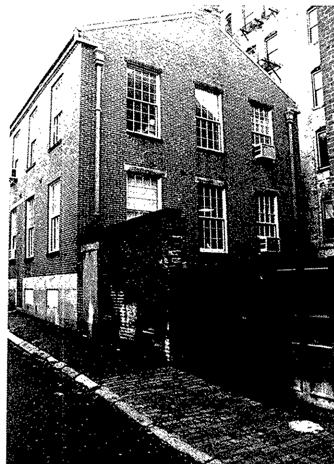
Figure 29. Smith School House: north and west elevations (1990).
