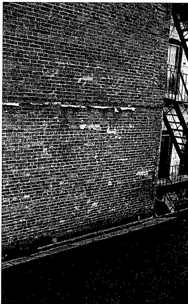
Figure 34. Smith School House: Junction of roof with adjacent south building, showing flashing line remaining from circa-1910 roof alteration (1990).
