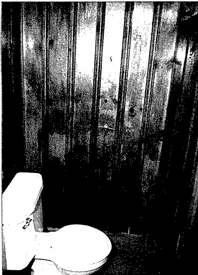
Figure 46. Smith School House: Cellar, men's toilet enclosure (1990).
