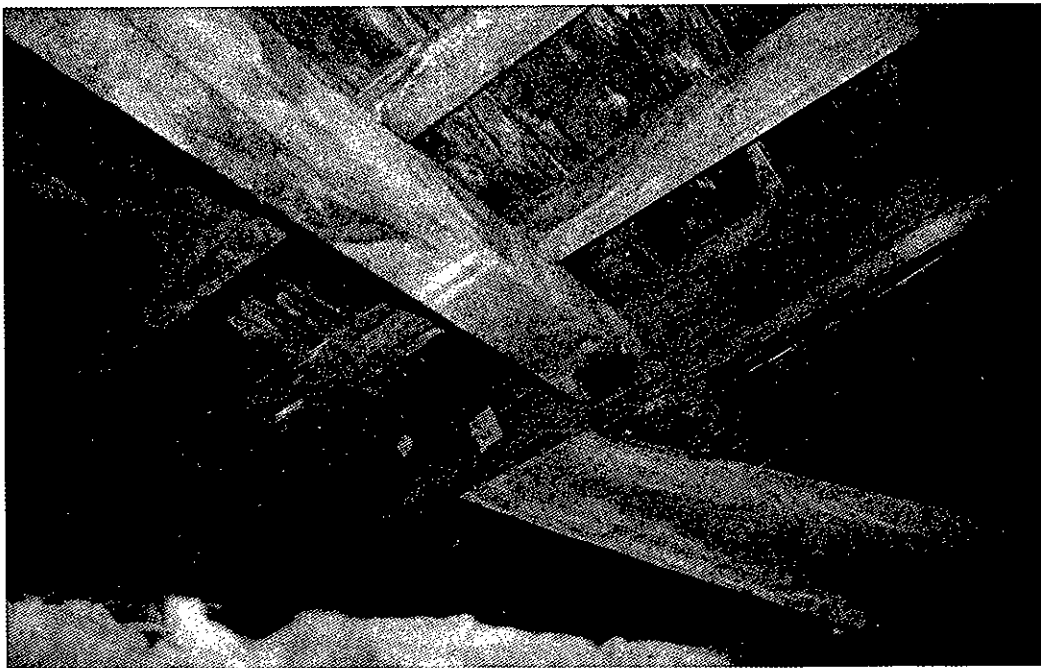
Figure 75. Smith School House: Attic, looking northeast at rafters and purlins (1990).
