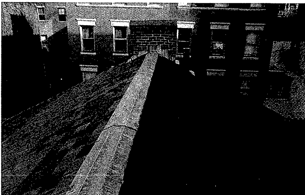
Figure 32. Smith School House: Roof, looking east (1990).
