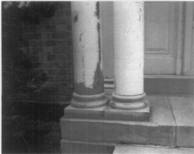
Figure 11. The lower shaft of the porch columns had decayed as water wicked up through the end grain (top). The column shafts were repaired in place by cutting out the deteriorated wood and making repairs using epoxy consolidants and fillers. (bottom). The column bases were replaced. Photos: Paul Marlowe, Marlowe Restorations.
