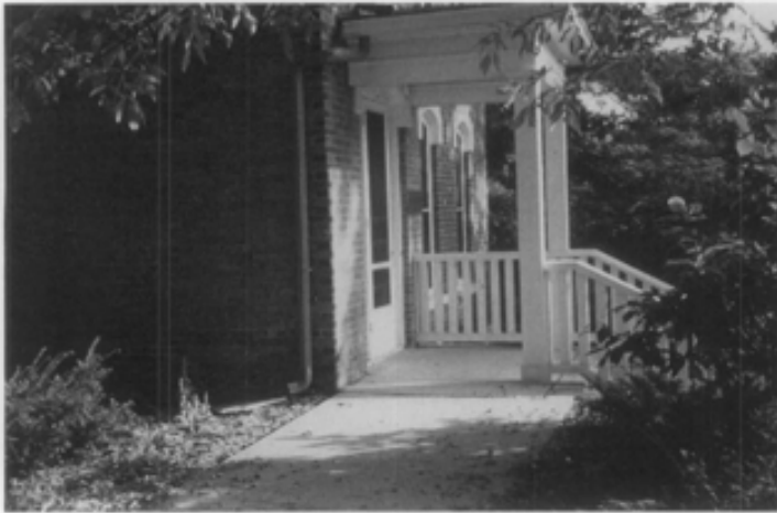
Figure 18. When a porch is used as a wheelchair accessible entrance, it may be possible to retain the historic stairs by adding a ramp parallel to the building. Through plantings and some re-grading, the new ramp built parallel to the building (left) allows retention of the historic stairs and does not impact the historic character of the entrance (right). Photo: Iowa State University Extension.
