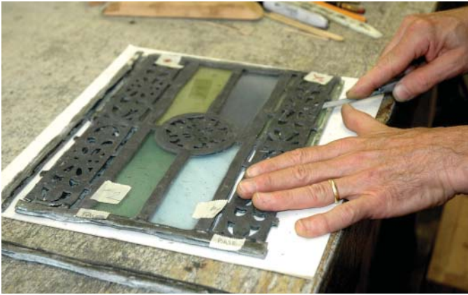
Figure 15. To permit repair of the cracked glass, the original lead overlay is first salvaged from this historic leaded panel of silhouette glass to retain as much of the original work as possible.
