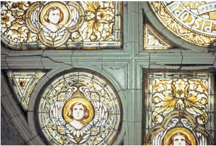
Figure 12. Stained glass frames are typically wood, steel or stone; however, other materials, and their inherent problems, can also be found as seen in this photograph of cracked terra cotta frames from 1926.
