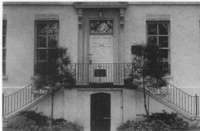
Figure 1. It is important to identify the materials, features, and spaces that should be preserved when planning accessibility modifications. These may include stairs, railings, doors, and door surrounds. Photo: National Park Service files.
