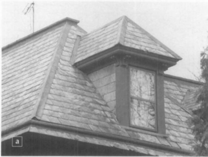
Figure 6. Hips are formed at the external angle of two roofing slopes. In (a), the hips at both the roof and the dormer are covered with metal. Note also the open valley and the built-in gutter. In (b), the dormer hip slates have been laid in a fantail pattern to help shed water. Note also the metal ridge cap.
