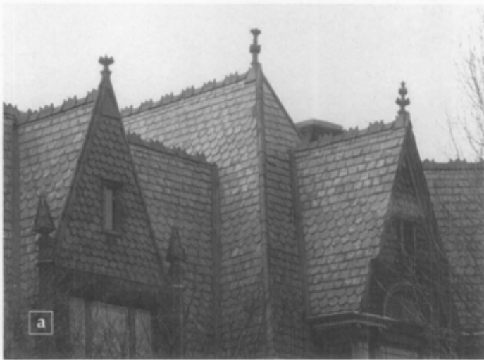
Figure 7. Ridge caps and cresting can be elaborate. Ridges are formed at the long horizontal juncture of two roofing slopes and capping protects this joint from moisture. In (a), a terra cotta capping with a decorative profile complements the finial over the various roof peaks. In (b), the mansard roof has a decorative iron cresting at the break between the lower and the upper roof slopes.
