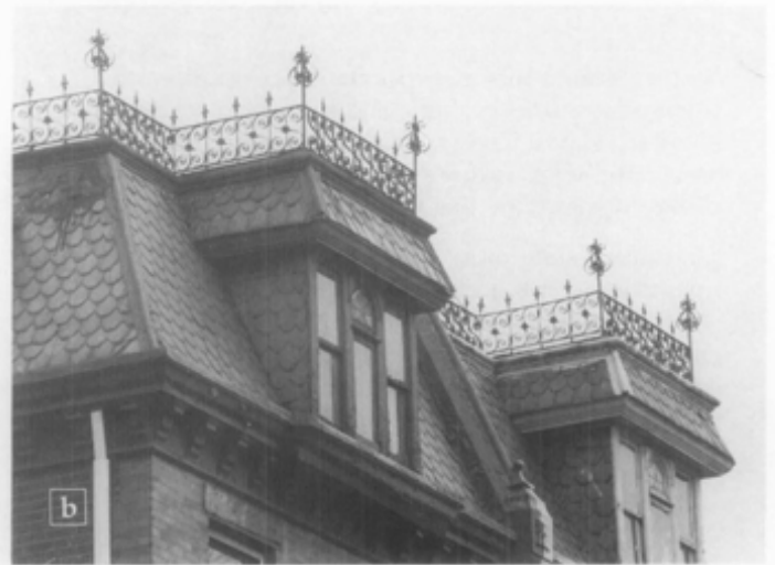
Figure 7. Ridge caps and cresting can be elaborate. Ridges are formed at the long horizontal juncture of two roofing slopes and capping protects this joint from moisture. In (a), a terra cotta capping with a decorative profile complements the finial over the various roof peaks. In (b), the mansard roof has a decorative iron cresting at the break between the lower and the upper roof slopes.
