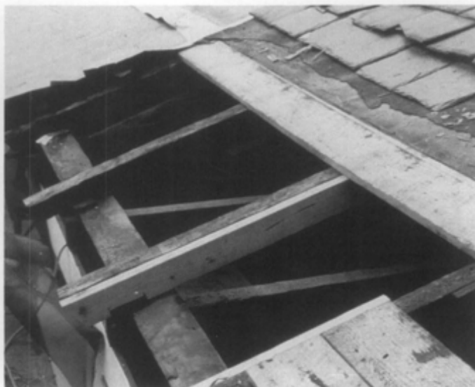
(d) Deteriorated sheathing was replaced and rafter tails were reinforced.
