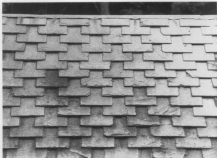
Figure 4. Widely spaced open slating was often used on utilitarian structures where ventilation was desirable. It provided an interesting texture and visual pattern to often plain structures.
