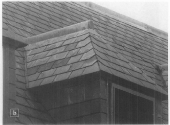
Figure 6. Hips are formed at the external angle of two roofing slopes. In (a), the hips at both the roof and the dormer are covered with metal. Note also the open valley and the built-in gutter. In (b), the dormer hip slates have been laid in a fantail pattern to help shed water. Note also the metal ridge cap.
