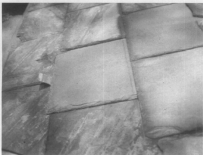
Figure 18. A method of securing replacement slates is shown. The copper strip is nailed to the roof sheathing just above the head of the slate in the course below. The replacement slate is then inserted and the copper tab folded over its tail. This type of repair is not recommended for northern climates where snow and ice can cause the copper tab to fold over, allowing the replacement slate to slide out of position as occurred here on the left.
