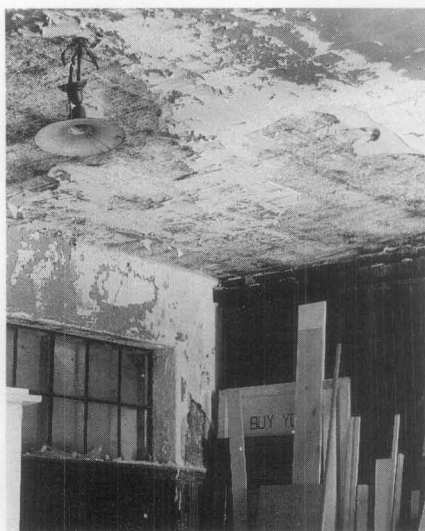
Figure 13. Part of a historic freight depot, this is not a high-style room and its painted surfaces are obviously in poor condition from long-term neglect. Interior spaces that are being converted for a new use in rehabilitation projects can benefit from being repainted in historic period colors rather than a neutral off-white. Photo: National Park Service files.
