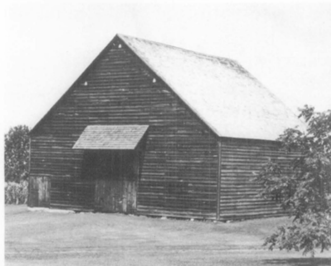
Built in the late 1700s, this New York Dutch barn survives in excellent condition. Gable roof, center wagon doors with pent roof, stock door at the corner and horizontal clapboarding are all typical features of the Dutch barn. Three holes for martins, traditional features of Dutch barns, can be seen near the top of the facade (they have been plugged and are lighter than the surrounding clapboards). Photo: Clarke Blair.
