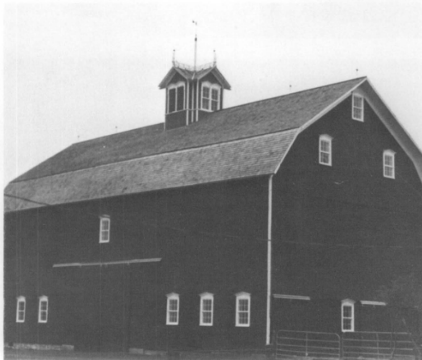
Fig. 8. Built in the Gothic Revival style in the 1890s, this four-story Indiana barn had fallen into disuse, and was deteriorating. In the process of returning it to use, the owner installed a new roof that matches the wooden shingles found beneath the deteriorating asphalt shingle roof; removed the modern asbestos shingle siding; repaired the windows, and reconstructed the cupola (including its lightning rod and weathervane). (Before and after views are of opposite sides of barn.) Photos: Before, Courtesy, Gary Post-Tribune; After, Courtesy, Kankakee Valley News.
