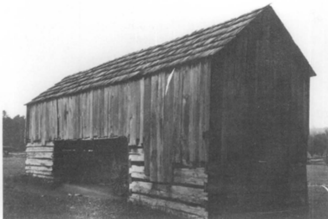
This late-nineteenth century crib barn is located in eastern Tennessee, in what is now the Great Smoky Mountains National Park. The central driveway between the cribs allowed a team and wagon to drive through after unloading. The materials and details are typical of the region. They include, on the exterior: hand-hewn saddle notched logs on the lower, crib portion; board framing on the upper, loft area; wood shingle roof. The interior features wood hinges on the crib doors and earth floor. Photo: Robert Madden.
