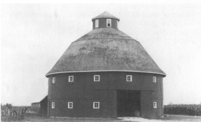
Circular barns are found throughout the country, but are especially numerous in the Midwest. This 1911 Illinois round barn is 60 feet in diameter. The cupola atop the hipped roof is 60 feet above ground. Its 10 single and 5 double stalls on the ground floor were fed from a loft. The square windows spaced at regular intervals around the perimeter add a note of simple contrast to the overall circular motif. Photo: Keith A. Sculle, Illinois Historic Preservation Agency.
