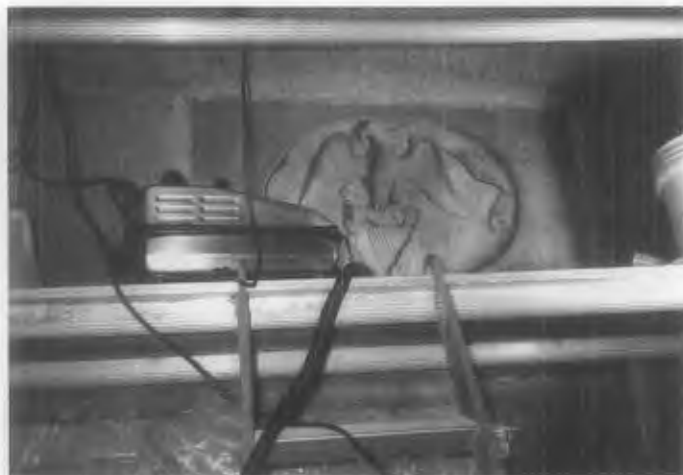
Figure 9. (Left) This small steam cleaner—the size of a vacuum cleaner—offers a very controlled and gentle means of cleaning limited, or hard-to-reach areas or carved stone details. (Right) It is particularly useful for interiors where it is important to keep moisture to a minimum, such as inside the Washington Monument, Washington, D.C., where it was used to clean the commemorative stones. Photos: Audrey T. Tepper.
