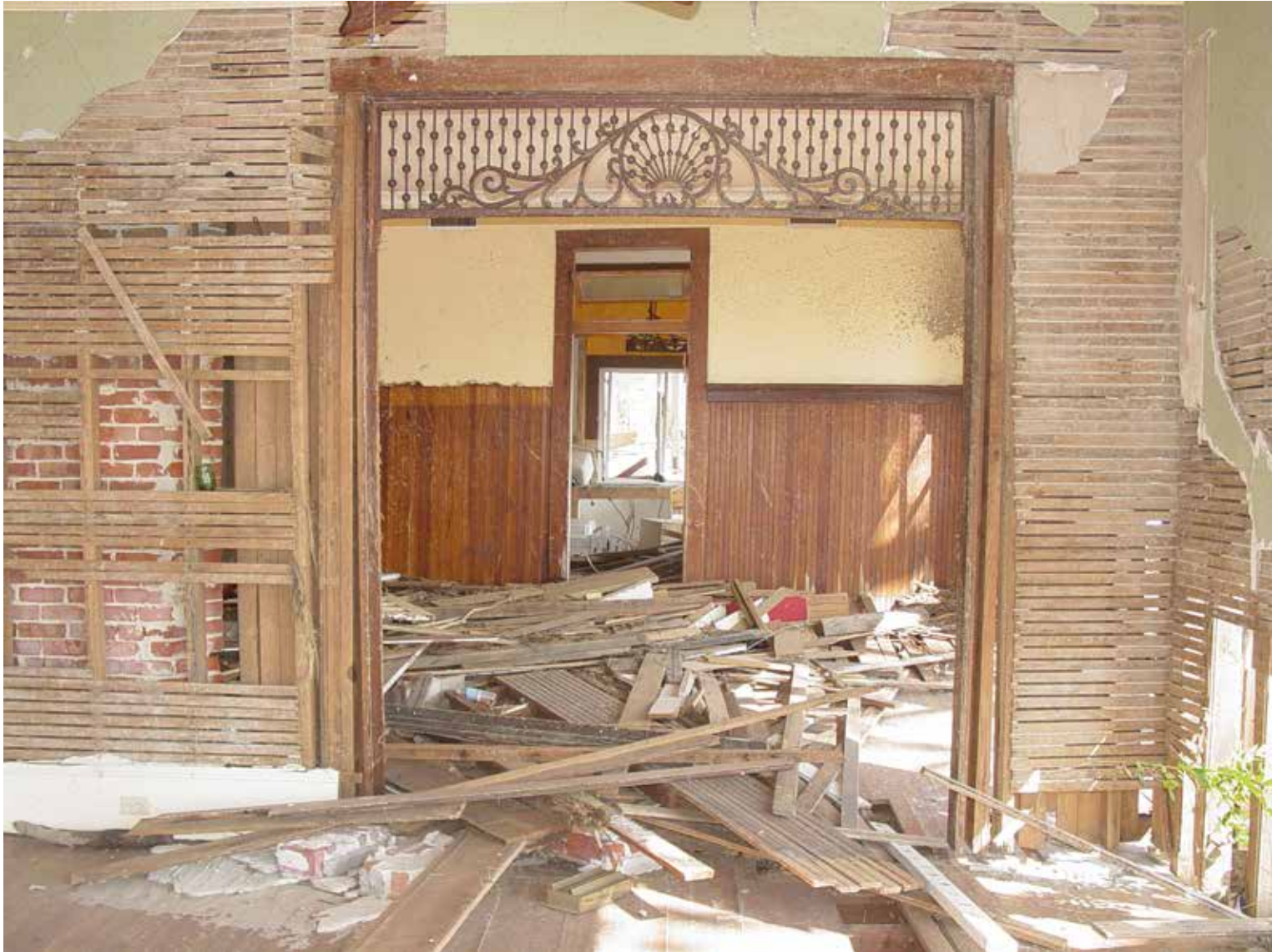
[6] Flood waters can also damage interior spaces. This historic home in Bay St. Louis, MS, was severely impacted by the storm surge from Hurricane Katrina. Even with such dramatic damage, it is crucial to properly assess the condition of historic materials and identify what remains and can be retained. In this case, most of the woodwork, the wood wainscot, upper sections of plaster in some rooms, and some areas of flooring were cleaned, dried, and repaired. Photo: Mississippi Department of Archives and History, Mississippi Historic Resources Inventory (HRI) Database. http://www.apps.mdah.ms.gov/Public
