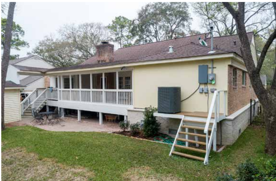
[44] Access issues must be considered when relocating exterior mechanical equipment on an elevated platform. If electrical or gas meters are moved to higher locations, stairs or a ladder may be required by the utility company to facilitate meter reading. Photo: p3elevation.com
