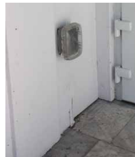
[61] This electrical box is protected with a removable waterproof plastic covering. Alternatively, electrical outlets can be located above the flood inundation level. Photo: Liz Petrella/NPS
