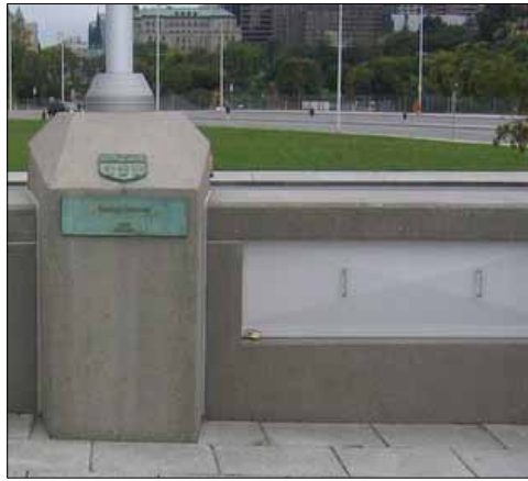
Standardized utility hookups can be disguised in bollards, reducing the need for temporary facilities. Shown are utility hookups in Ottawa (left and center) and a utility bollard in Chicago's Millennium Park (right).
