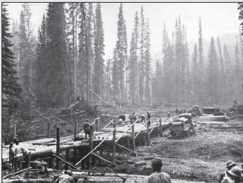
Black engineers build a trestle bridge during the construction of the Alaska Canada Military Highway. Black G.I.'s made up roughly forty percent of the estimated 11,500 Army troops who in just nine months completed a wilderness highway linking Alaska with the contiguous United States. (Anchorage Museum of History and Art)
